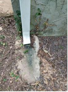
Recommend gutter downspouts be extended and routed away from the building atleast 4-6ft. for proper drainage. Water seepage into crawl spaces, basements and under foundations can be caused by inadequate removal of rainwater from the perimeter of the house.
