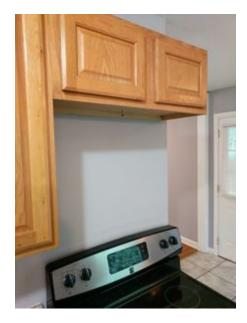
No exhaust fan was observed. Today's construction would require installation of a fan / hood.
