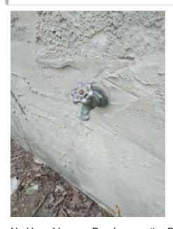
No Hose Vacuum Breakers on the Outside Hose bibb at the time of inspection.
