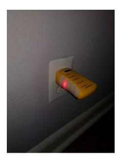
Three pronged outlets did not test for proper ground. For Safety add atleast (one) GFCI outlet to every room and connect all other outlets to it in the each room with improper ground. Normally this is every room. Label with (NO EQUIPMENT GROUND) on the outlets. Recommend further evaluation and repairs by a licensed electrician.
