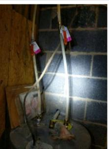
PEX is the main water supply to the water heater. Normally Copper is at least present 18in before PEX or other materials are allowed. It is suggested that a "Licensed Plumbing Contractor" be contacted for further evaluation and correct.
