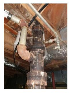
Galvanized piping was observed. Although this type of piping was commonly used in older homes, galvanized piping is no longer used in today's construction. Galvanized piping has a tendency to rust from the inside. This condition can reduce the water flow and pressure.
