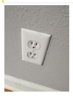
Some outlets were painted over. These outlets should be replaced.
