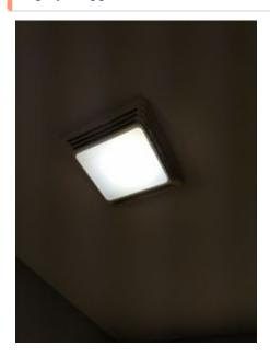
Vent /Vents were covered by insulation in the attic space.
