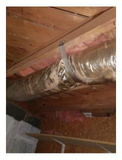
Evidence of condensation building up in the ductwork/register notice. This could be current or in the past. The inspector is unable to confirm this.
