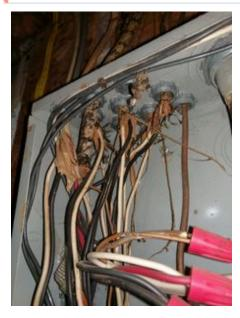
Some cloth covered wire insulation was present. Although installation and usage of this wiring was typical at the time of installation, today's construction no longer uses this out dated wire insulation. Client is advised to consult with a licensed electrician for further information.
