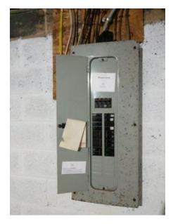
Rust / corrosion was observed at the panel box or breakers. Recommend further evaluation by a licensed electrician.
