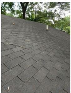
The roof showed advanced signs of aging and deterioration. This condition can indicate imminent leakage. Replacement is recommended. Recommend further evaluation by a qualified roofing contractor. The inspector cannot offer an opinion as to whether the roof leaks today unless it is moderately raining at the time of inspection. Client should obtain full disclosure / history information from the seller prior to close.
