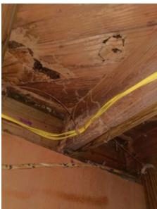
Evidence of wood damaging insects. Possibly a past infestation I would recommend a pest inspection to determine if it is active.
