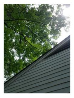
Tree branches / leaves were close to or in contact with roof surfaces. Recommend trimming branches back to prevent potential roof damage.
