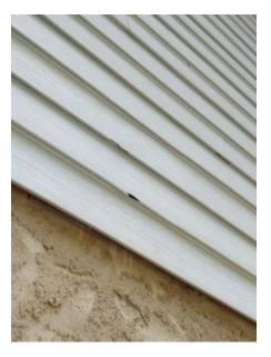
Chipped / Cracked siding was observed. Seal/Repair or replace if needed the siding to prevent water from entering behind the siding.
