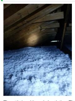
The attic has blown-in insulation. The approximate depth of the insulation is 10+ inches, which appears adequate.
