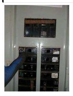
The panel and some of the breakers inside the panel do not match.
